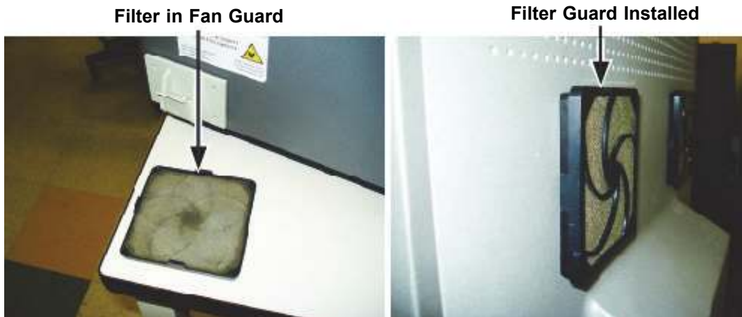
Figure 9-13. Replacement Filter and Guard Installed
