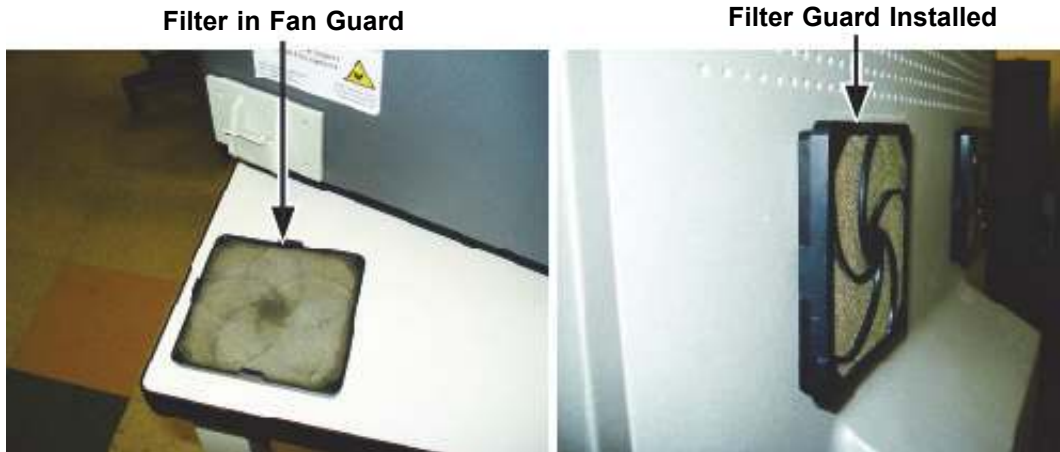
Figure 9-13. Replacement Filter and Guard Installed
